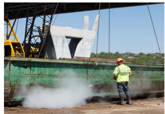
Figure 2. Removal of aquatic remnants is required before transporting.
