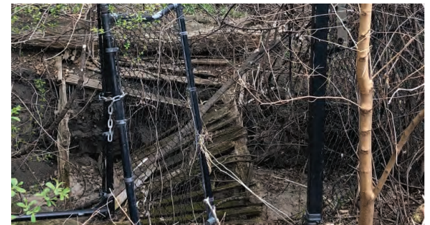
Access from the Boardwalk apartments easement is restricted with fencing and a collapsed bridge.
