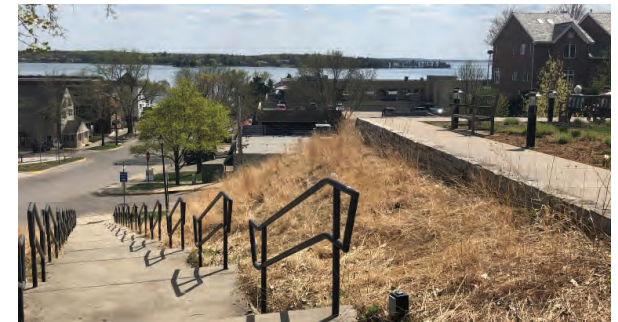
Existing Stairway leading to Lake Street
