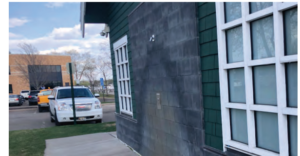
Existing showers hidden behind the building.
