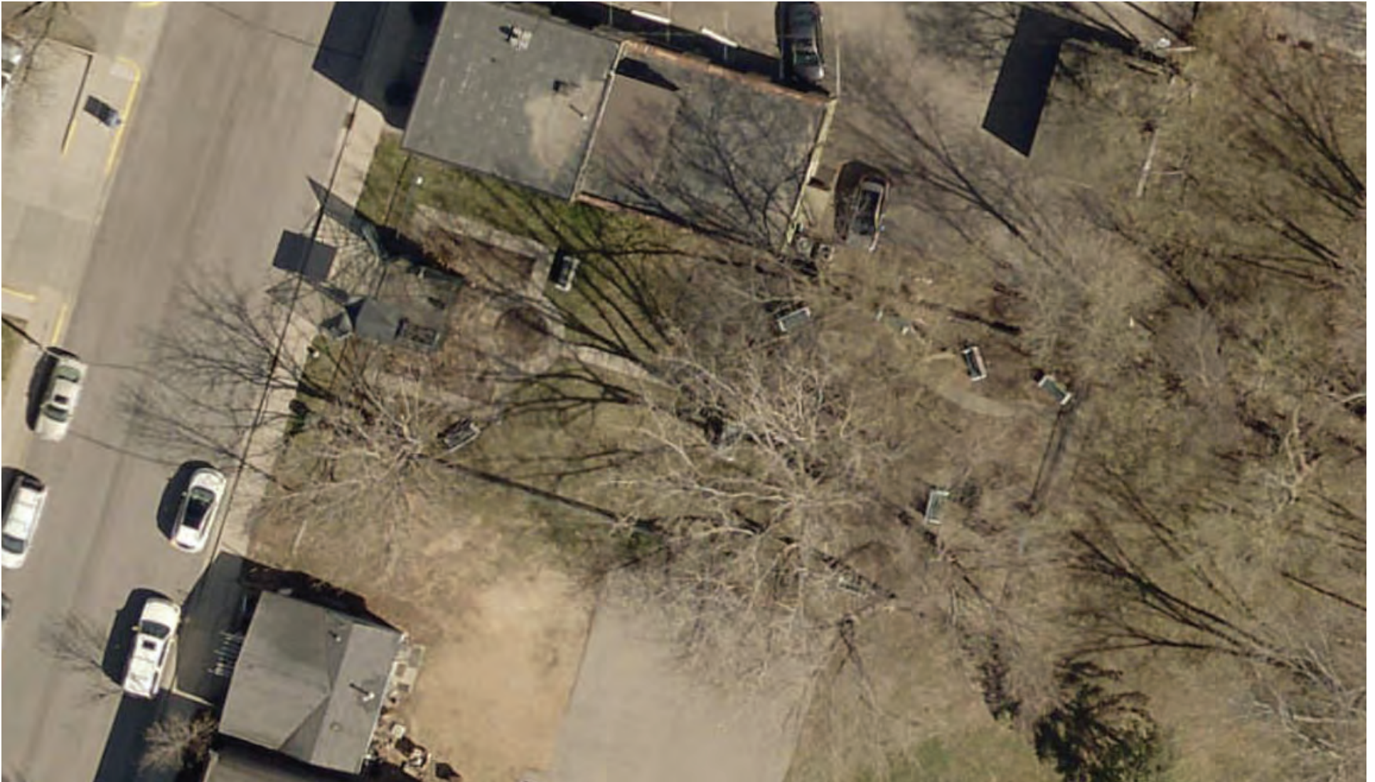
POST OFFICE POCKET PARK EXISTING CONDITIONS
